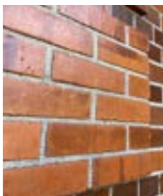
Sealed Brick Exterior
